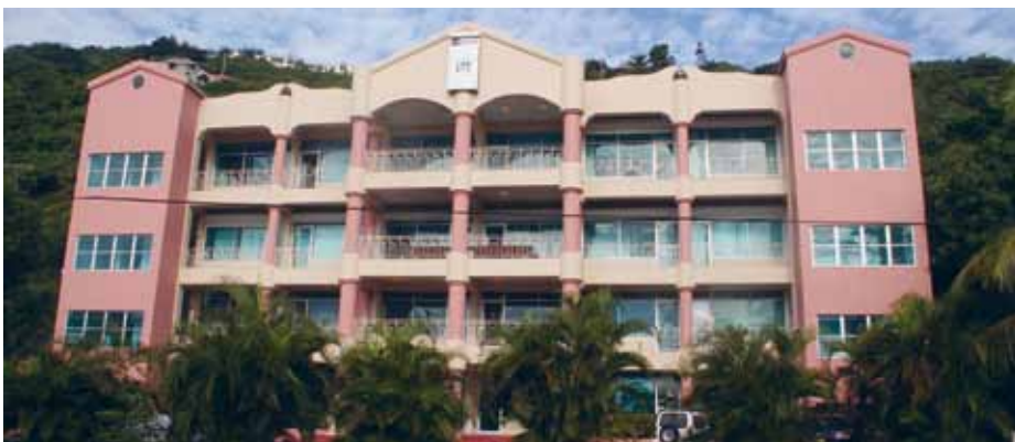
Gebäude von ATU General Trust (BVI) in Road Town, BVI
